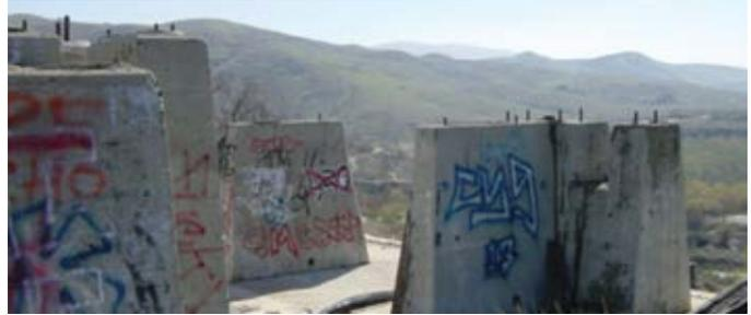
The concrete from the old structure on the abandoned mine site at Dos Lagos development was crushed and used as base material for Temescal Canyon Road.
